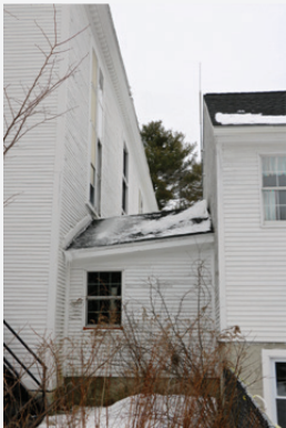
Replaces old connector & its poor water/snow management
