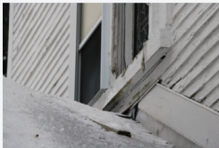
Replaces old connector & its poor water/snow management
